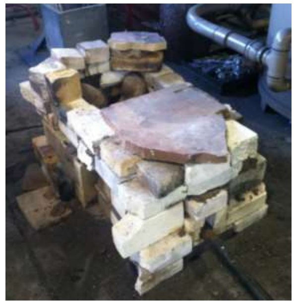
The flue at the back of the kiln.
