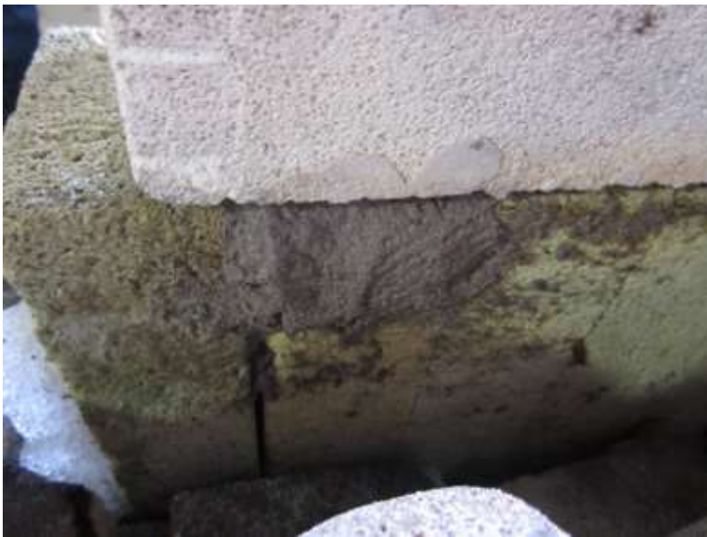
The tuyere left for the pipe to fit into.
